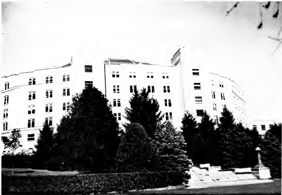
This scene shows the main entrance of West Baden College, revealing the picturesque surroundings of the pleasant Indiana countryside.
